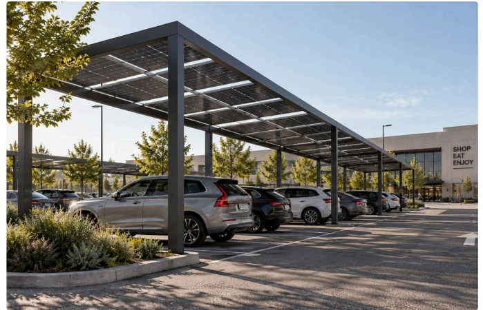
PHOTOVOLTAIC SHADING PERGOLA
